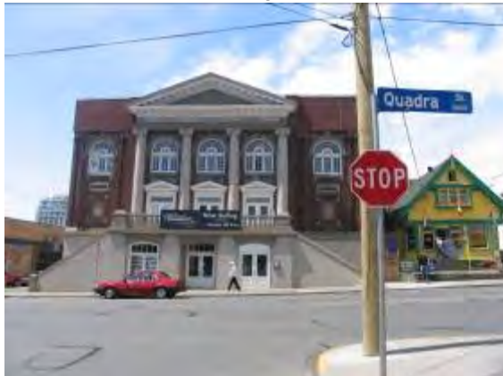
Palladian Building at a Street Head
