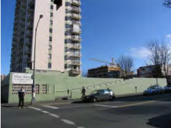
Blank Parkade Structure Walls
