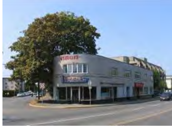
Richmond Road, Birch and Fort Street Intersection
