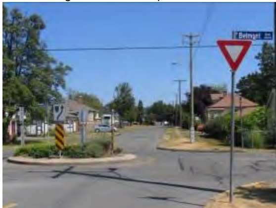
Kings Road Landscaped Traffic Circles
